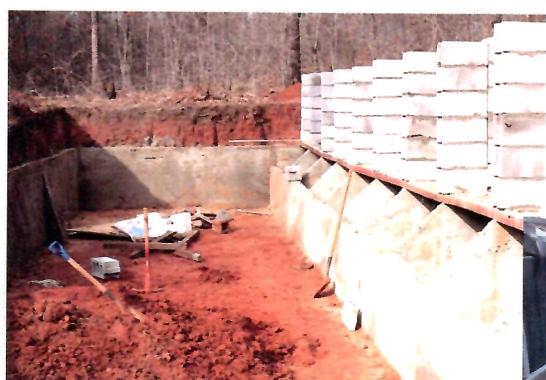
Above: Detail of the construction of partially buried vivaria. This is a major project involving careful consideration of the orientation of the vivaria and careful planning in the construction - the benefits will warrant the efforts.
